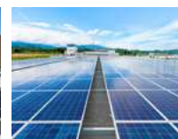
Solar power generation facility (Tohoku site)
