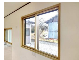
Example of installing double-paned window
