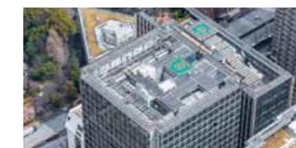
Solar power generating equipment on the roof of the IINO Building
