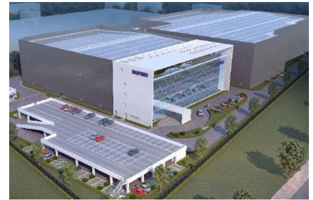
A new plant for cleanroom systems (Suzhou, China) will introduce a rooftop photovoltaic system in 2023.
