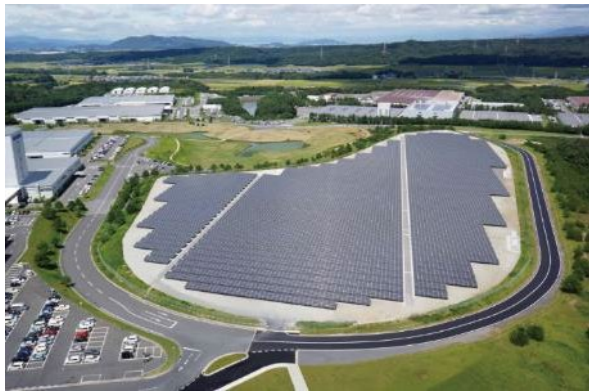
Mega solar farm at the Shiga Works operating since 2013
