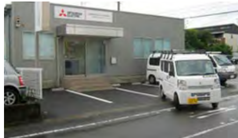
Repair Service Station(2)
