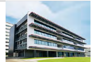
ZEB testing facility "SUSTIE"
