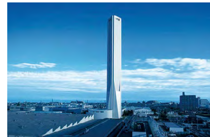
SOLAÉ elevator testing tower
