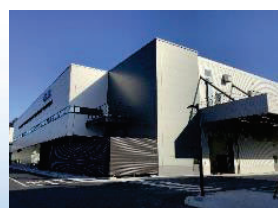
Kamaishi No.5 Plant
