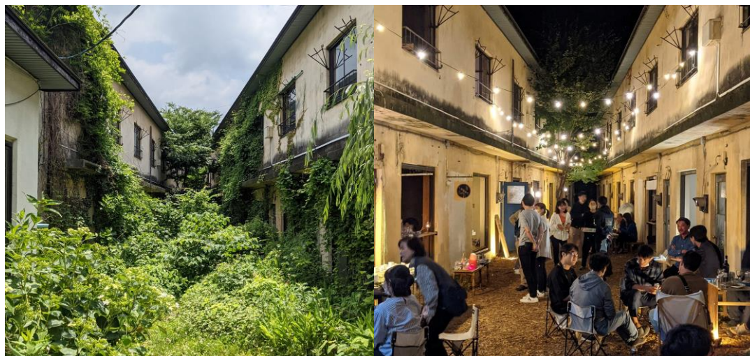
Before the maintenance
