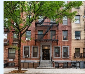
Value-up building appearance
