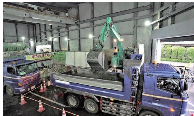
Trial autonomous operation of a power shovel.
