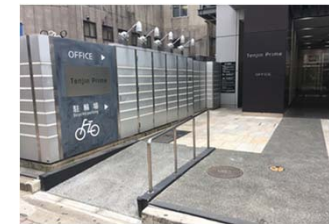
Barrier-free renovation construction (Tenjin Prime)
