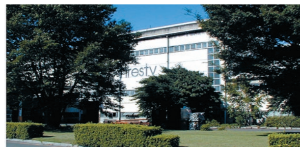
Kumagaya Plant with plenty of greenery
