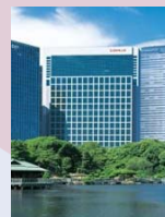
Tokyo Shiodome Building
