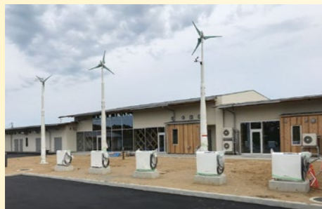
MICHINOEKI (Roadside Station) NAMIE—Site of Information Dissemination Green EV system connected to renewable energy
