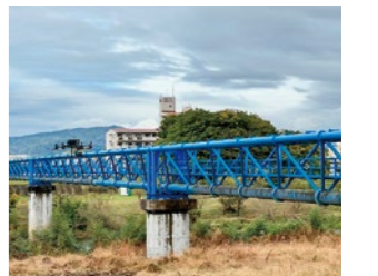
Inspecting a water pipe bridge using drones
