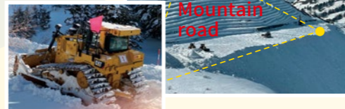
Case: Construction machinery safety enhancement model, in Gunma
