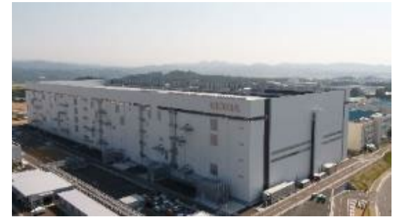
Kioxia Iwate Corporation Kitakami Plant
