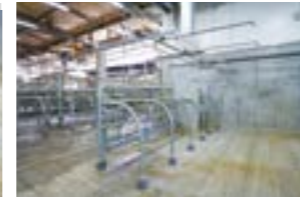
Berthing facility with misting system
