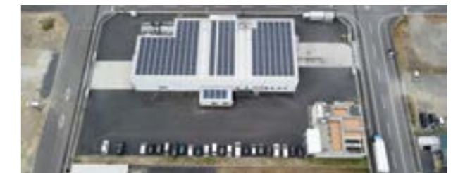
Solar power generation system at SMP Akune Plant Processed Food Production Center
