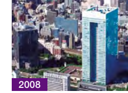
2008 NREG TOSHIBA BUILDING joined the Group
