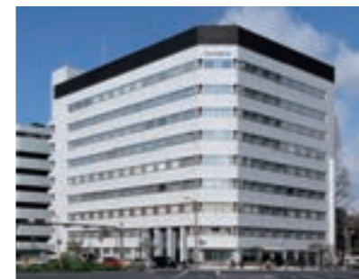
Shinmachi 1 Building (Completed in 1988)
