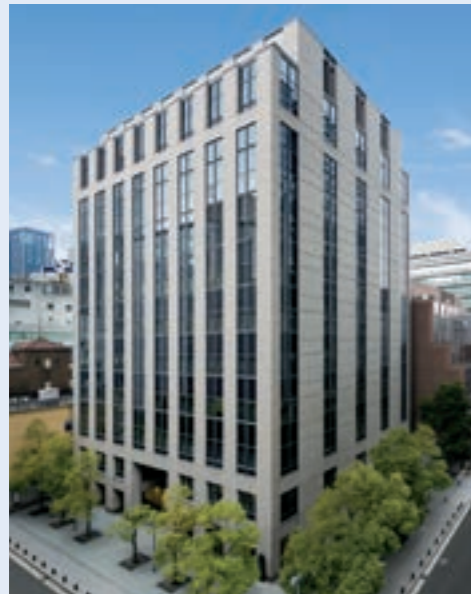
Keihanshin Yodoyabashi Building
