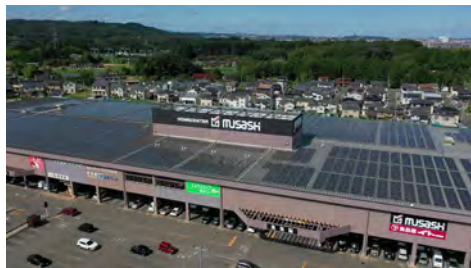
Industrial solar power system
