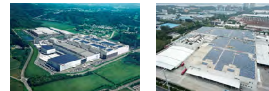
Solar power systems installed on the roofs of Sharp production bases (left: Kameyama Plant; right: NSEC in China)
