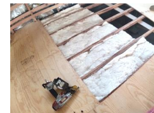
Example of installing insulation
