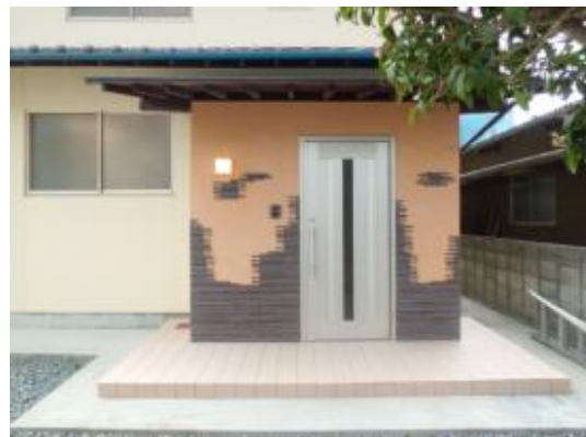
House where porch tiles were replaced, a new exit door was installed and the exterior wall was clad with accent tiles
