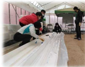
Covering the bed with waterproof, water supplying, and root barrier sheets, and spreading pumice on top of the sheets
