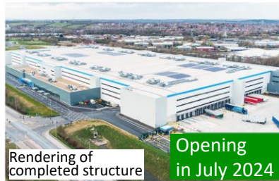
Opening in July 2024 Kanto New Distribution Center (26,100m 2 ) 513 Minaminagai, Tokorozawa city, Saitama
