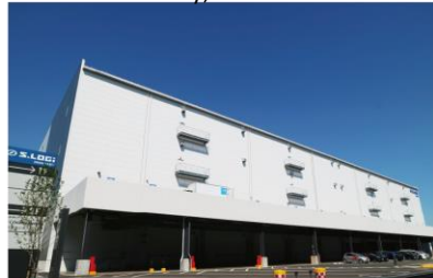
The 3rd Tokyo Distribution Center (9,300m 2 ) 3-3-21 Owada, Niiza city, Saitama
