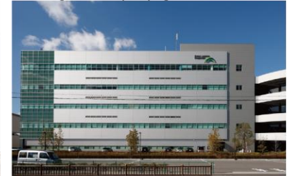
D-to-C II Distribution Center (13,200m 2 ) 231-2 Nishimukojimacho, Amagasaki city, Hyogo
