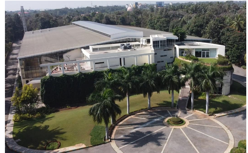
▲ View of the new factory
