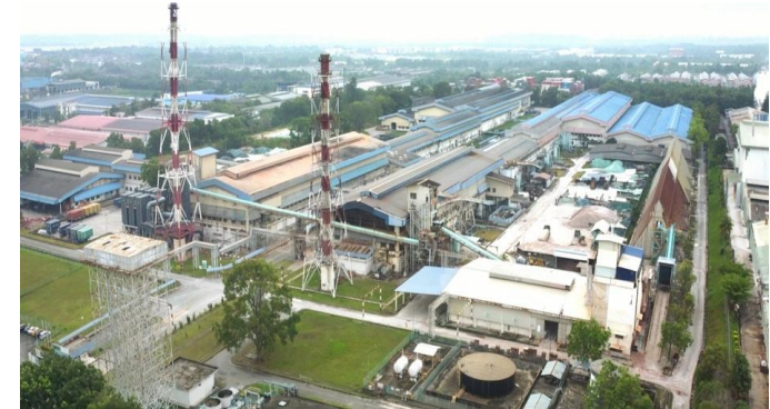
Float furnace in Malaysia
