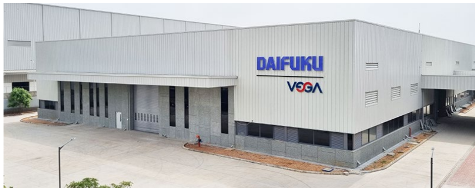
A plant currently in operation
