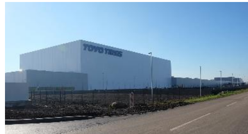
Panoramic view of the plant
