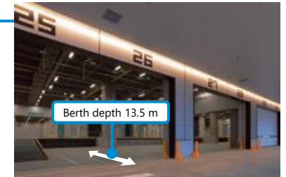
Truck berths are large enough to fit a whole 40ft container truck.
