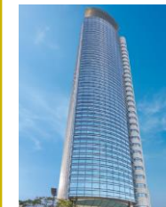
Nakanoshima Mitsui Bldg. (Osaka City, Osaka)
