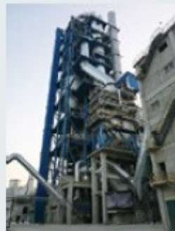
Cement plant waste heat power genera- tion facilities
