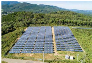
Creation of renewable energy by solar fund
