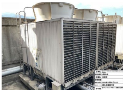
Before removal of old cooling tower
