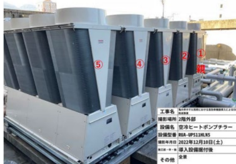
After installation of air-cooled heat pump chiller
