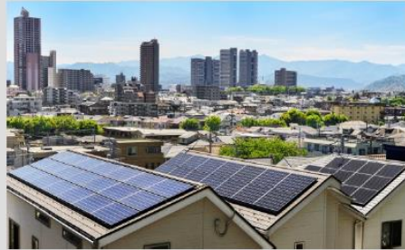
The Tokyo Metropolitan Government making the installation of photovoltaic panels mandatory
