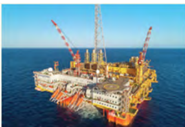
Offshore production and central processing facility (CPF)
