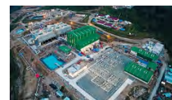
Muara Laboh Geothermal Power Plant
