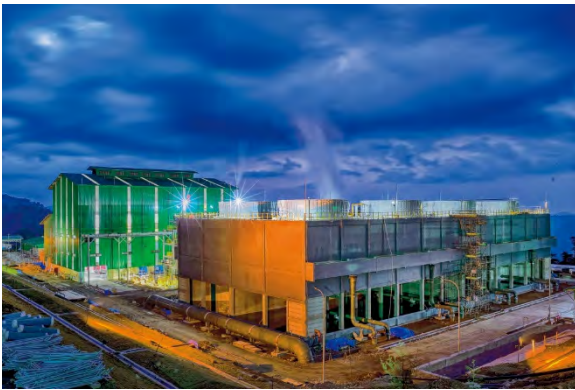
Muara Laboh Geothermal Power Plant
