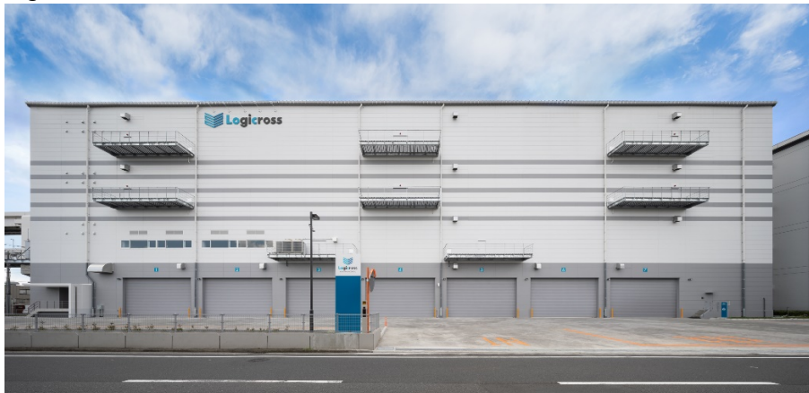
Logicross Yokohama Kohoku
