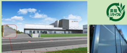
Soundproof wall with Soundproof Panel containing used tea leaves at Toyo Mebius Kumagaya Logistics Center.
