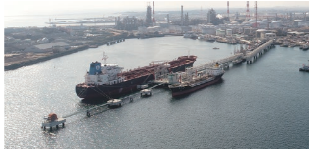
Reinforcement of marine jetty with a view to strengthening disaster response capabilities (Yokkaichi Refinery of Showa Yokkaichi Sekiyu Co., Ltd.)
