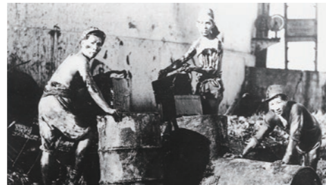
Collecting oil from the bottom of a tank
