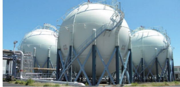
LPG tanks with reinforced support structures (Tokuyama Complex)
