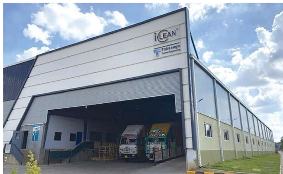
Exterior view of the new plant
