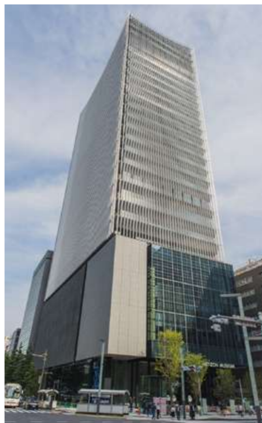
Realization and demonstration of an open-plan skyscraper for Museum Tower Kyobashi Received the 36th Award for Promotion of Technology from the Society of Heating, Air-Conditioning and Sanitary Engineers of Japan
