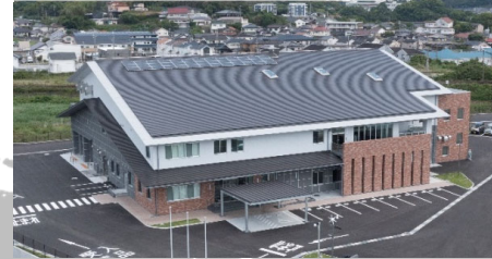
Sludge Recycling Plant
