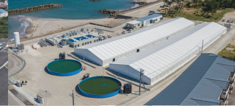
Onshore Aquaculture Plant (Water Treatment System)
