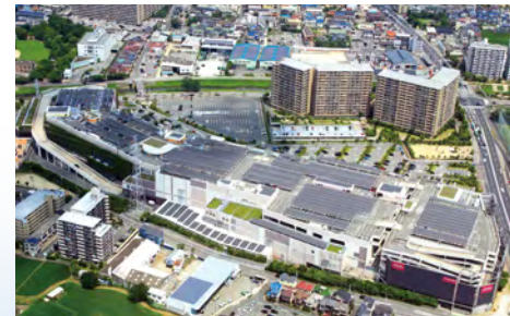
Solar panels installed on the rooftop and walls help reduce the environmental burden
