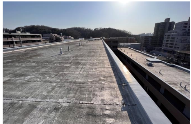
Rooftop where solar power generation equipment will be installed
