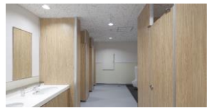
Installing water-saving toilet system
