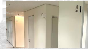
Common area signage
