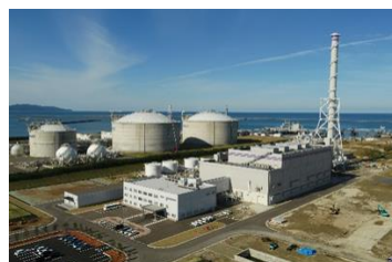
Joetsu Thermal Power Station
