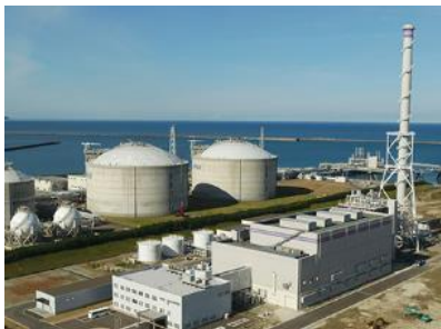
Joetsu Thermal Power Station
