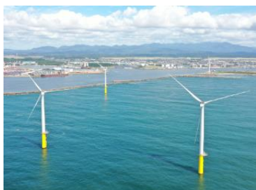
【Akita and Noshiro Port Offshore Wind】 Output 138,600kW (Operation Date:Jan.31 2023) Japan's first commercial large-scale offshore wind power project
