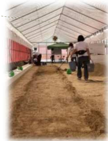
Digging a trench for the bed and leveling the ground
