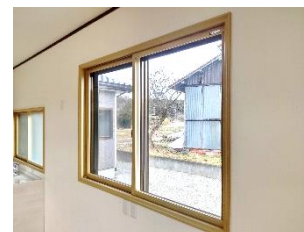
Example of installing double-paned window
