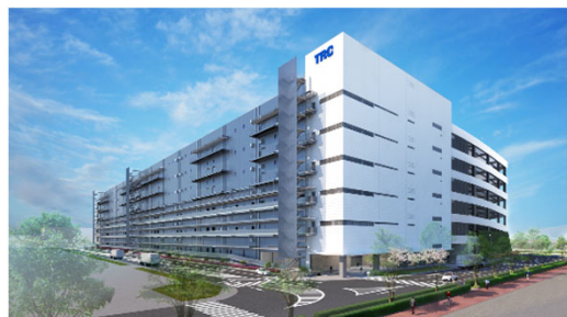
Tokyo Ryutsu Center Distribution A Building
