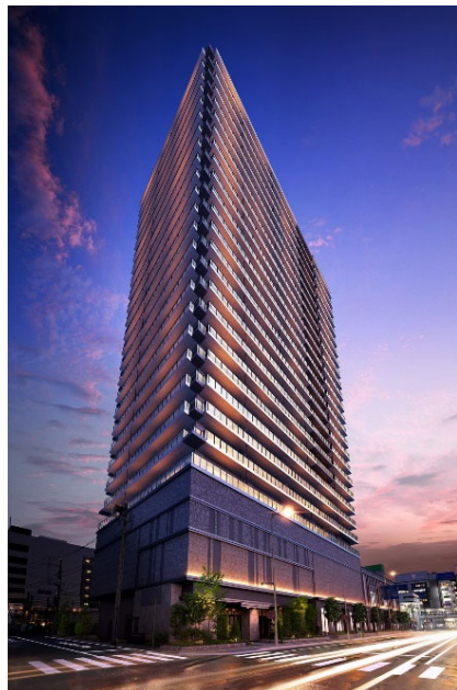
The Parkhouse Kawagoe Tower
