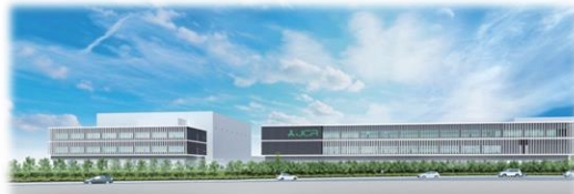
New formulation building (To be completed in 2027)
