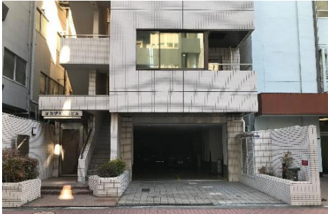
First floor was a dark parking area.
