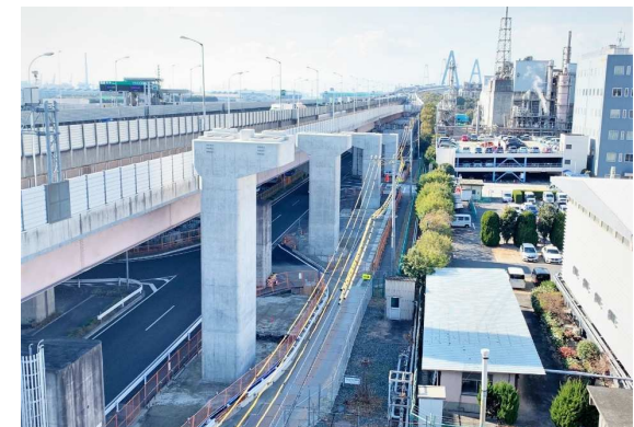
FY2020 Route 247 Nishi Chita Doro Tokai JCT/H Lamp Bridge Lower Part Project Tokai City, Aichi Pref. Client: Chubu Regional Bureau, Ministry of Land, Infrastructure and Transport
