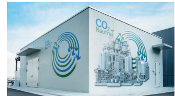
CO2 Circulation Plant
