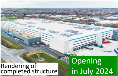
Kanto New Distribution Center (26,100m 2 ) 513 Minaminagai, Tokorozawa city, Saitama
