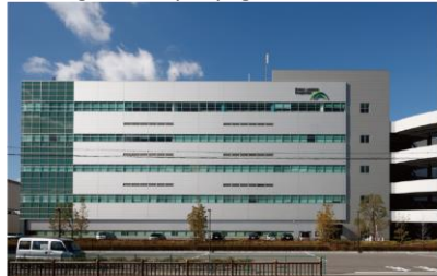
D-to-C II Distribution Center (13,200m 2 ) 231-2 Nishimukojimacho, Amagasaki city, Hyogo
